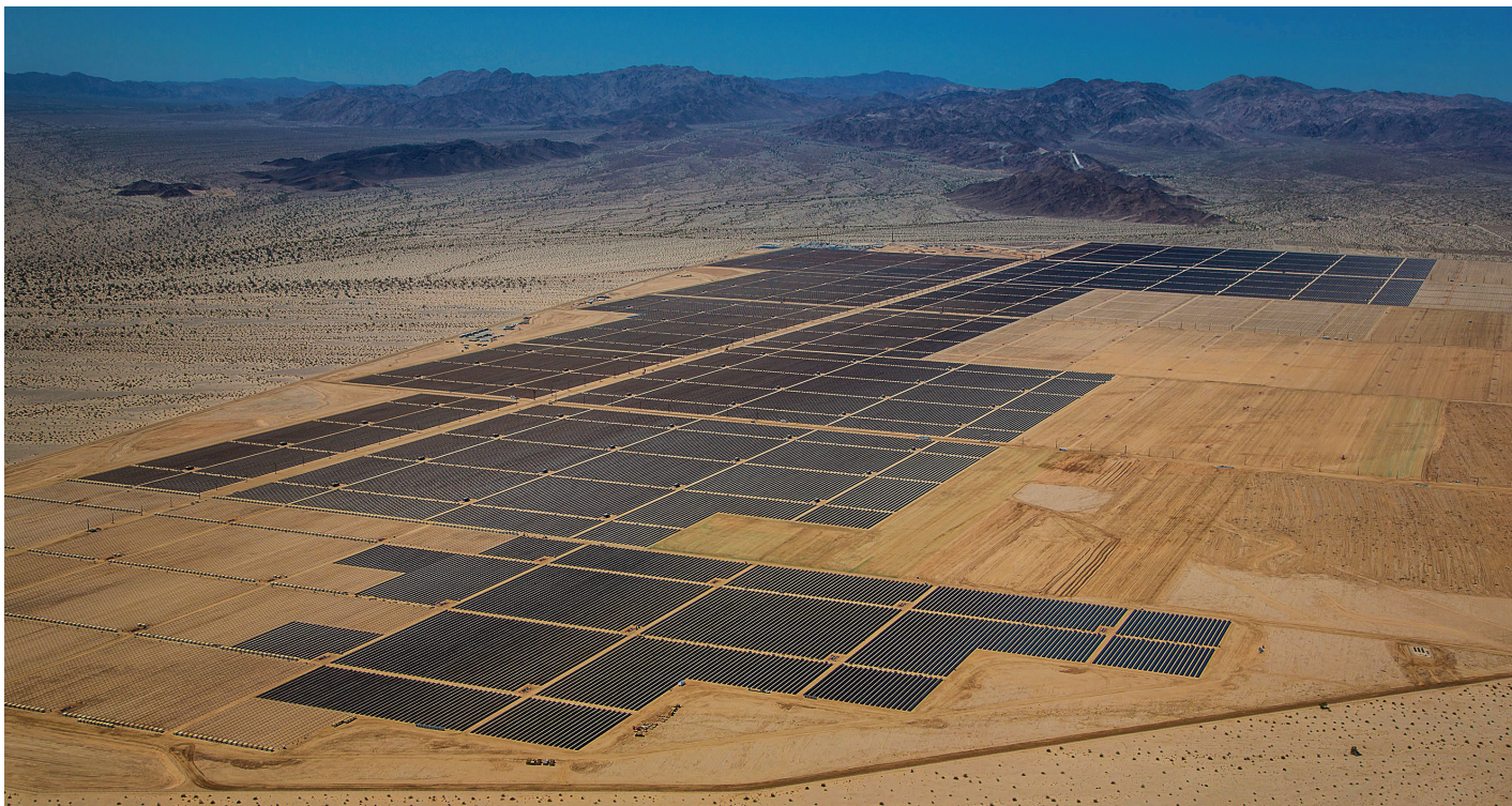
Topaz Solar Farm
